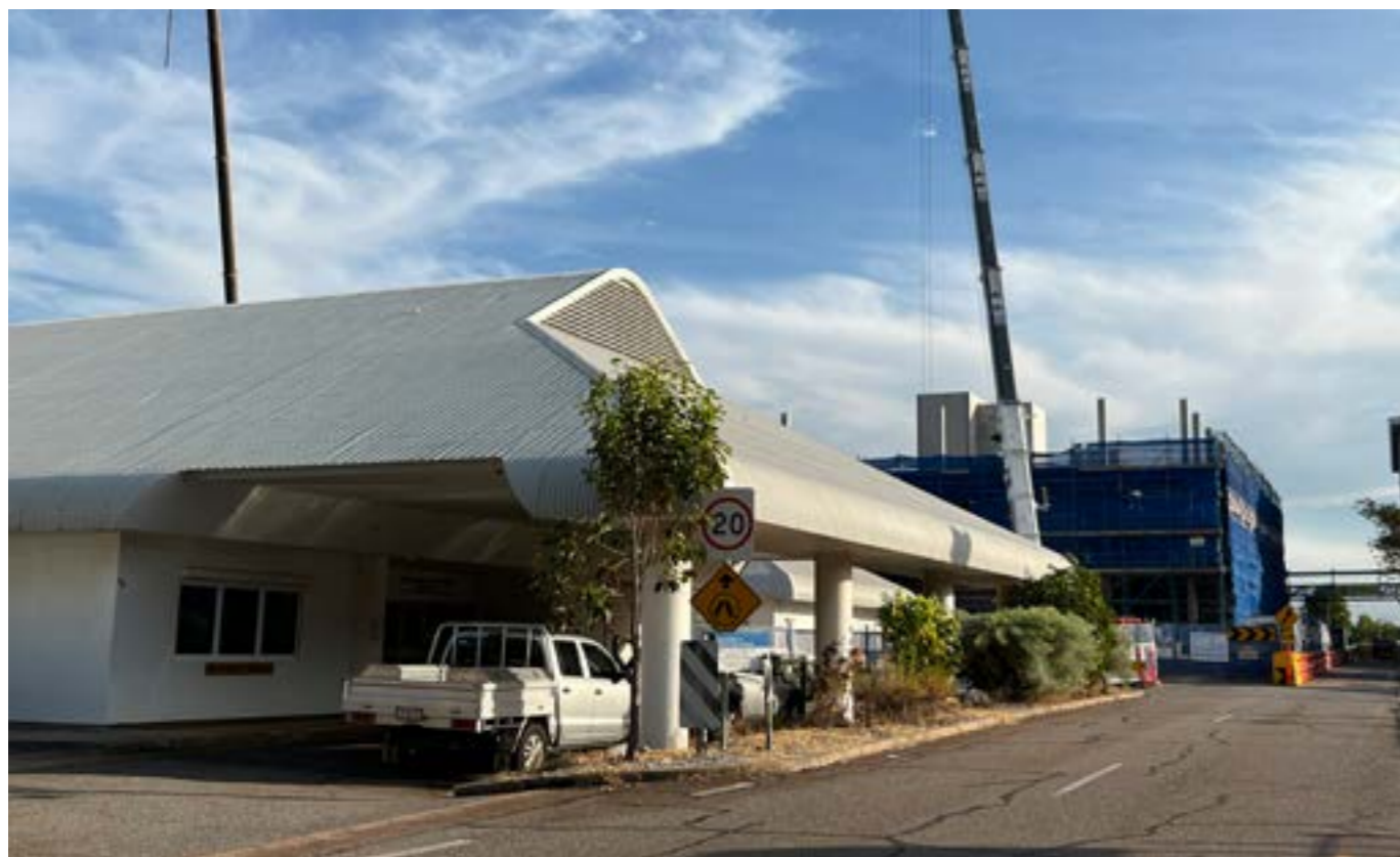
The 'new build' mental health facility adjacent to the IPU at RDH
